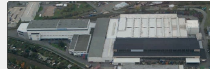
▲ A view of the Tower International plant in Zwickau
